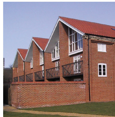
New housing based on former warehouses
