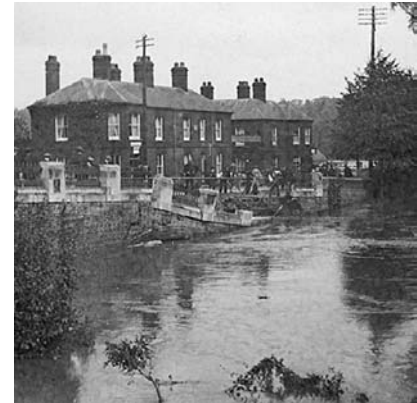
Collapse of bridge in 1912 © Norfolk County Council
