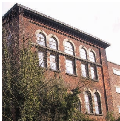
Trowse pumping station
