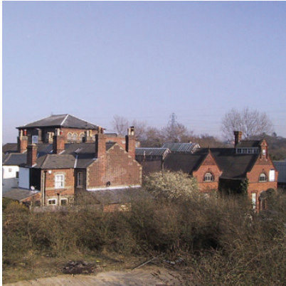
The pumping station rises above chimney stacks giving this part of the conservation area a very industrial feel
