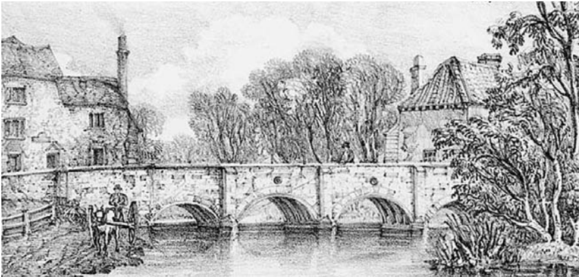
Trowse Bridge early 19th century © Norfolk County Council
