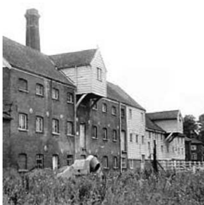
The mill in 1965 before demolition
