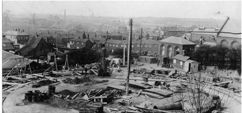
Construction of gas holder Gas Hill c1900. Photograph ©Norfolk County Council
