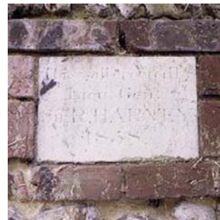
Plaque dated 1858 on the garden wall of 28 Telegraph Lane West
