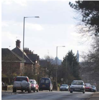
Views looking south along Constitution Hill toward the city centre.
