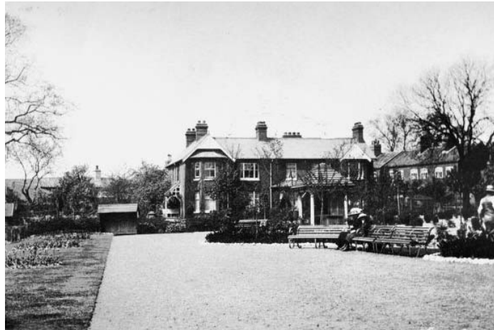
Sewell Park, north end looking west
