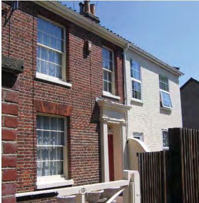
Loss of architectural details can significantly change the appearance of a building.
