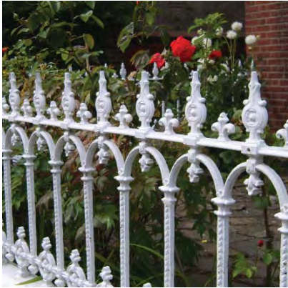
There are fine examples of late Victorian railings along Clarendon Road.
