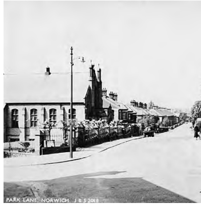
Former Methodist Church, Park Lane. (© Norfolk County Council)
