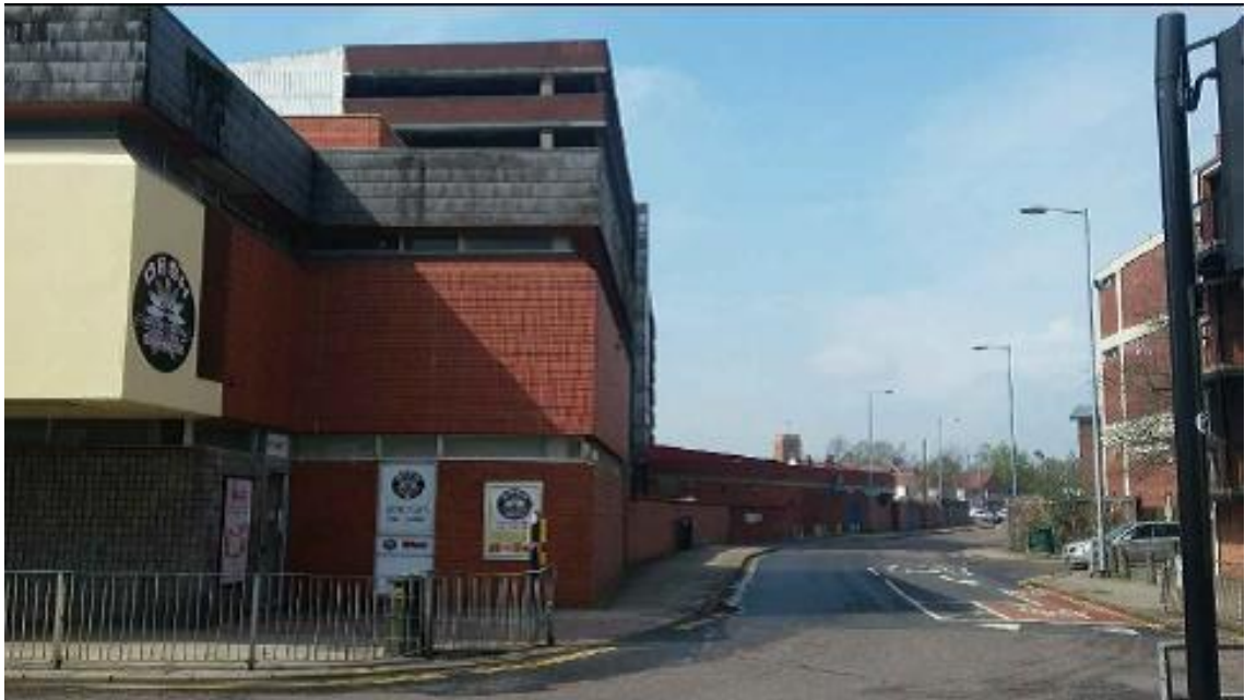
Northeast Boundary of Site Looking Along Edward Street
