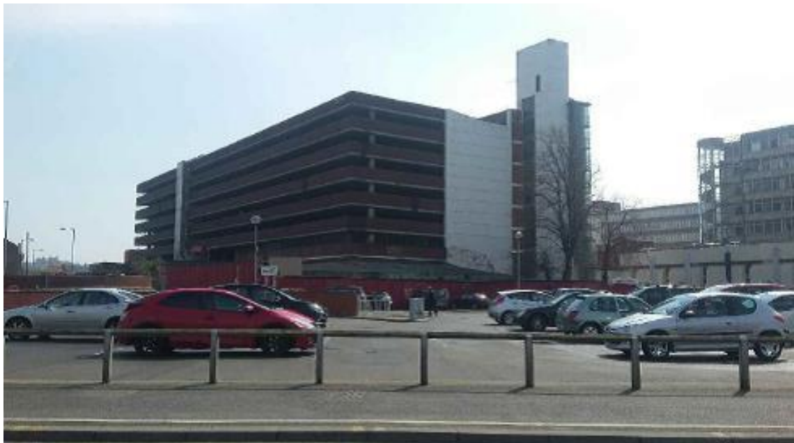
Multistorey Car Park and Northern Car Park
