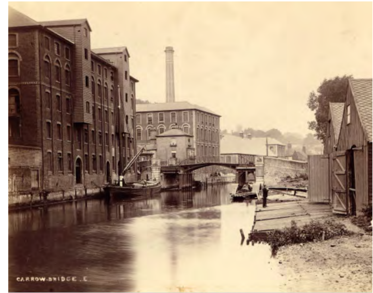
The original alignment of Carrow Bridge on the axis of Carrow Road - this opening bridge built in 1833 itself replaced an earlier fixed bridge - Image courtesy of www.picture.norfolk.gov.uk
