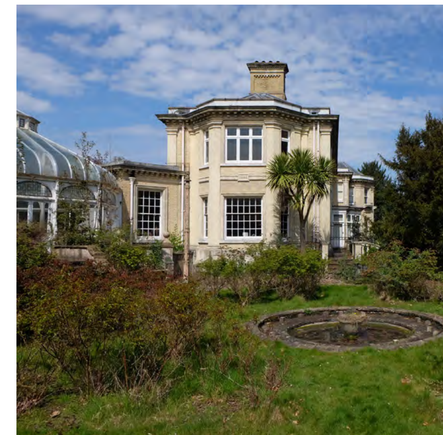
Grade II Listed Carrow House with adjacent conservatory and formal gardens
